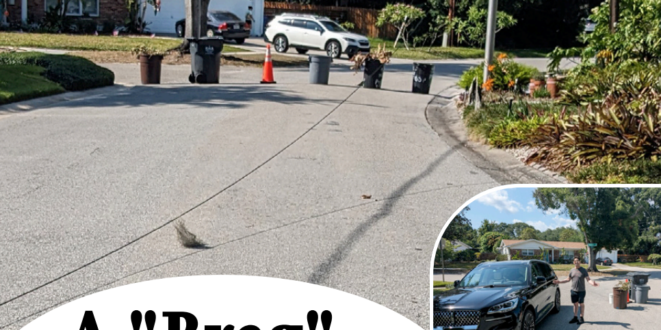
Downed line - 3" inches off of the ground in the middle of the street...still attached to power poles at both ends.
