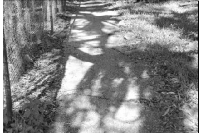
Before: Walkway behind Bank of America
